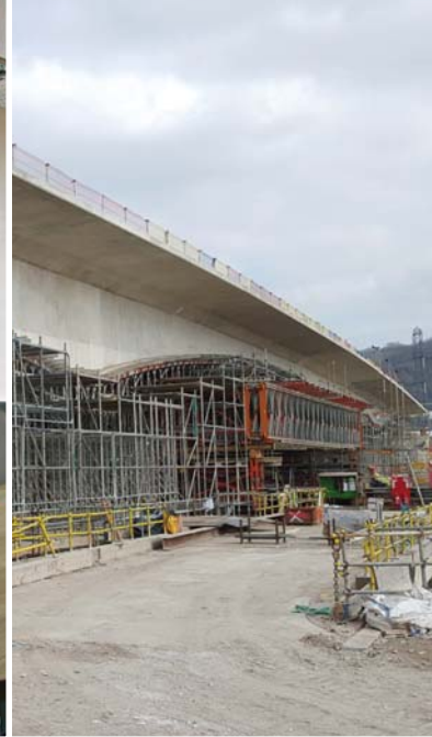
Medway River Bridge.
