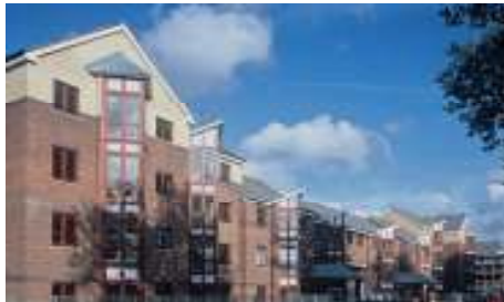
Nightingale Estate, Hackney, which use the high thermal mass of ready-mixed concrete together with passive solar design
