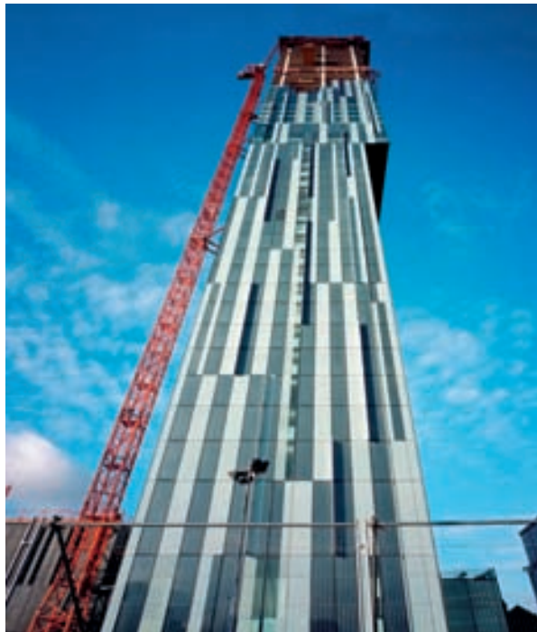
Specialist concrete contractor - MPB Structures
