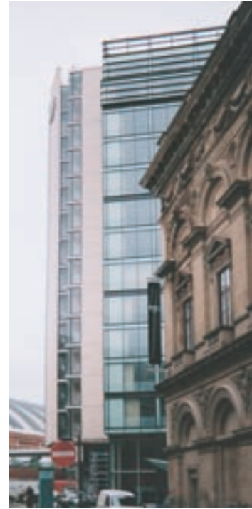
The new tunnel form Radisson Hotel behind its historic façade.
