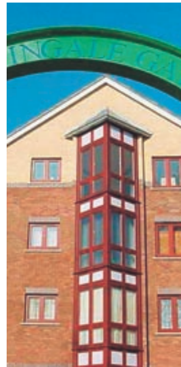
Shared ownership flats at the Millennium project, showing the bay windows achieved by modifying the formwork.
