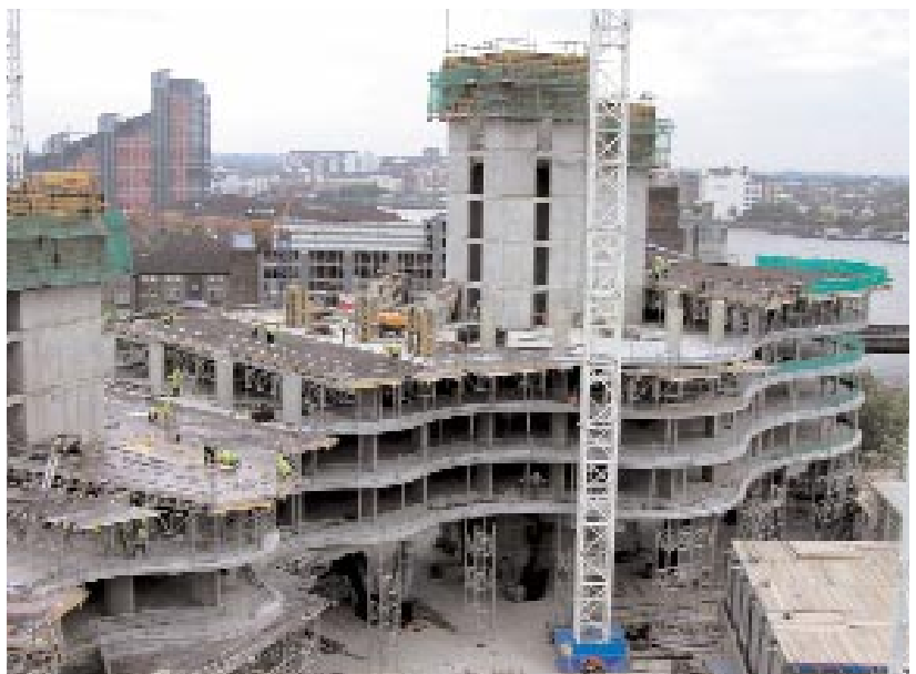
Figure 5: The core construction preceded the superstructure floors.
