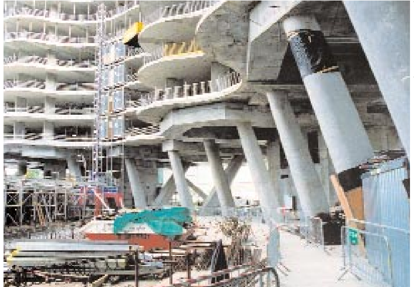
Figure 1: The V-columns separate the substructure from the superstructure.
