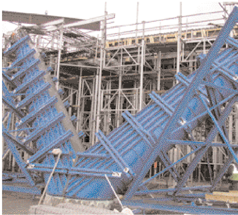
Figure 3: V-column formwork in position.
