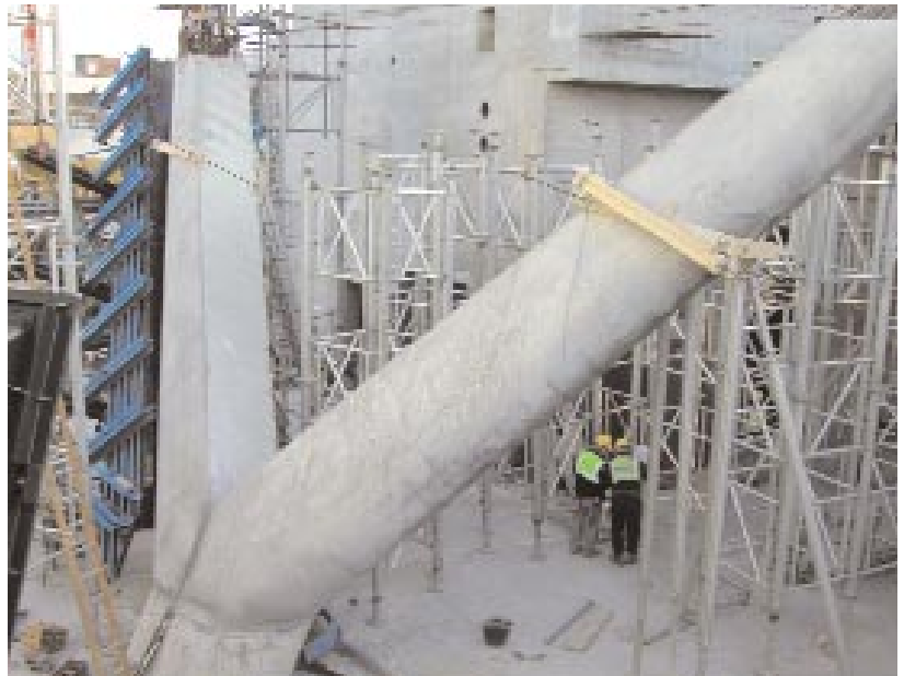
Figure 4: A high-quality finish was achieved on the concrete V-columns.
