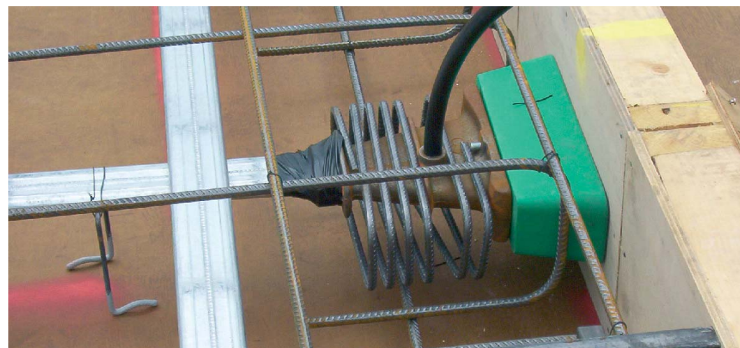
top left AMS House showing bonded PT slab with conventional reinforcement over columns and at construction joints. Specialist subcontractor Freyssinet Ltd.
